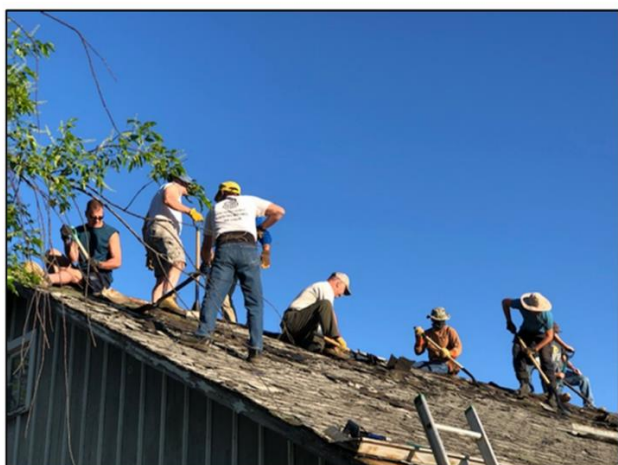
Removing a barn roof in Nebraska City
