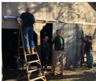
Installing siding and doors in Nebraska City
